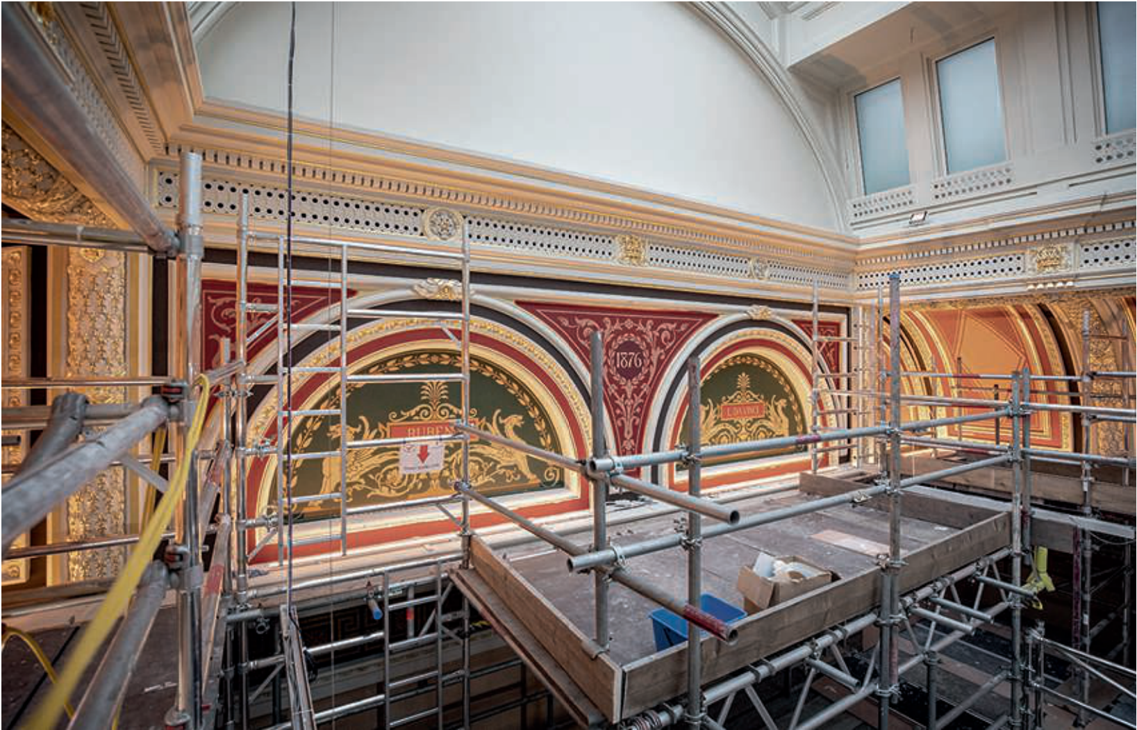
Installing the lunettes
