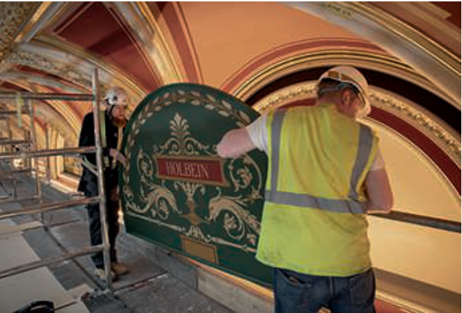
Installing the lunettes
