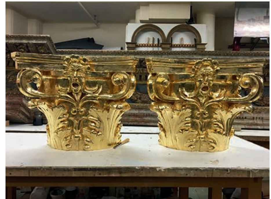
Gessoed capitals with yellow and red bole (above). The capitals are gilded prior to toning (below).
