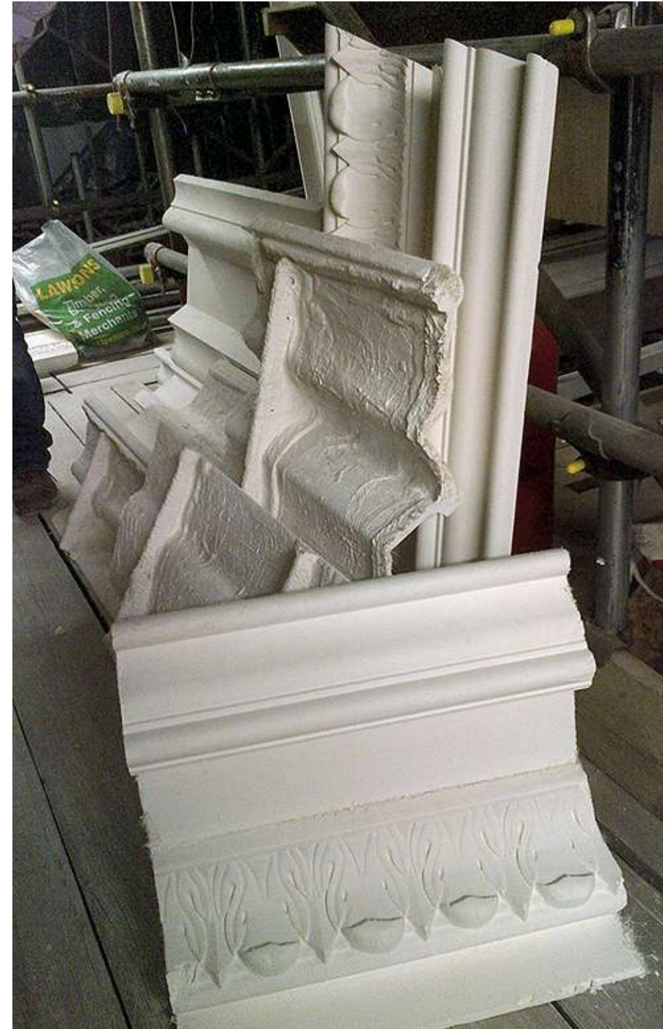
Opposite The application of plaster of Paris in Room 33
