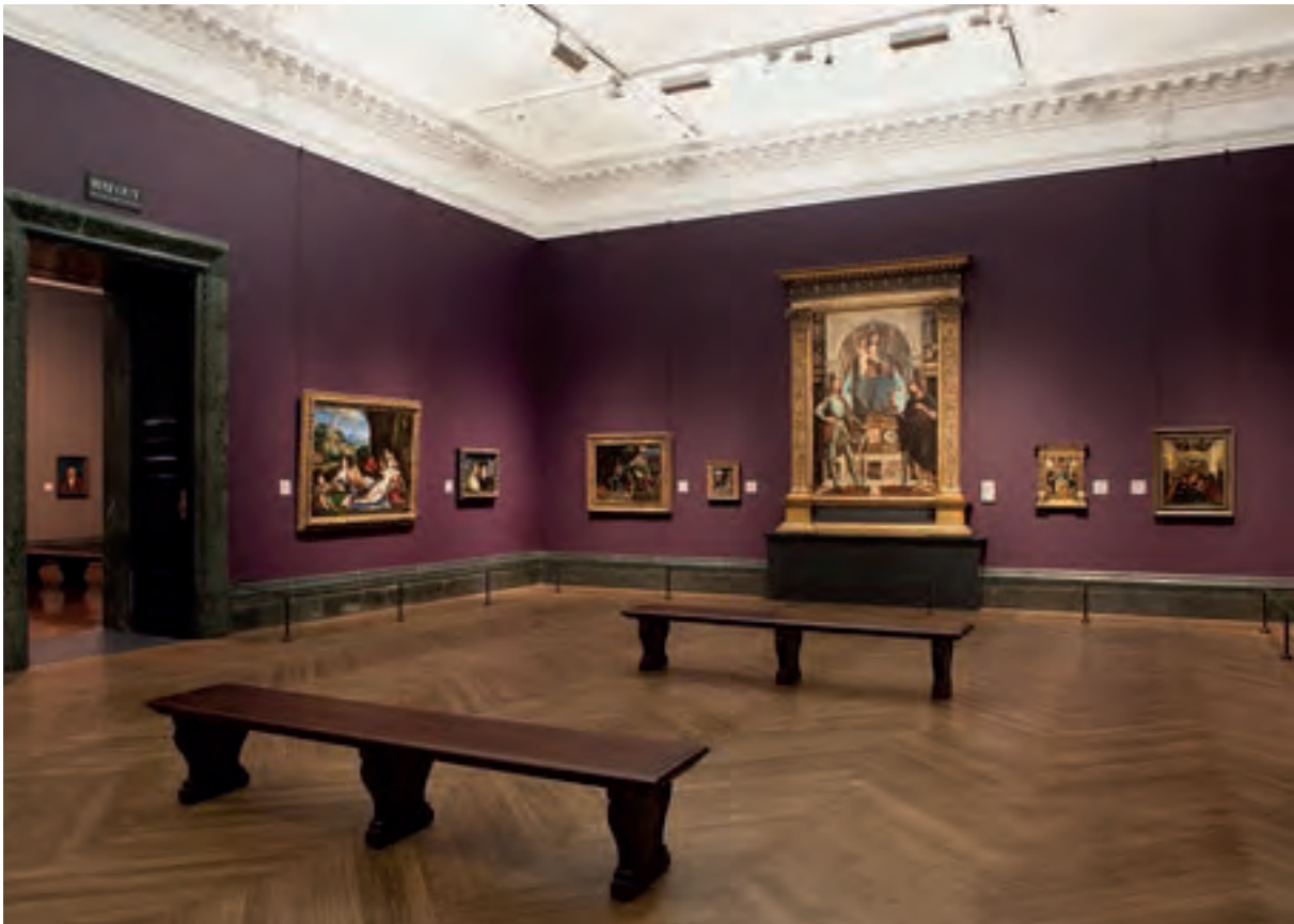
The new LED lighting installed in Room 6
